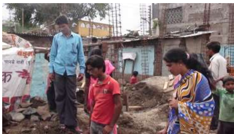
AMBEDKAR NAGAR. MAHILA MILAN CONTRACTOR MONITORING CONSTRUCTION 2011 JULY
